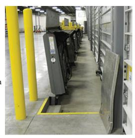
Although a number of companies offer vertical dock levelers, facility managers should consider a variety of specific features before committing to an installation. Most importantly, look for a "drive-thru" application that allows trailer doors to be opened inside the facility. Opening and closing trailer doors inside the loading dock, rather than on the drive approach, allow loading dock staff to place or remove the trailer's seal from inside the building—maintaining supply chain integrity.
