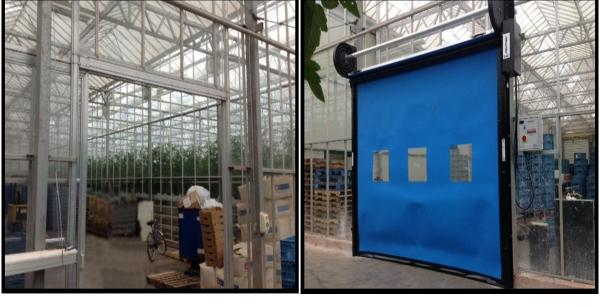
The Challenge: A way to section off the loading dock from the rest of the facility in order to maintain a certain level of humidity and temperature to ensure the successful ripening of tomatoes.
