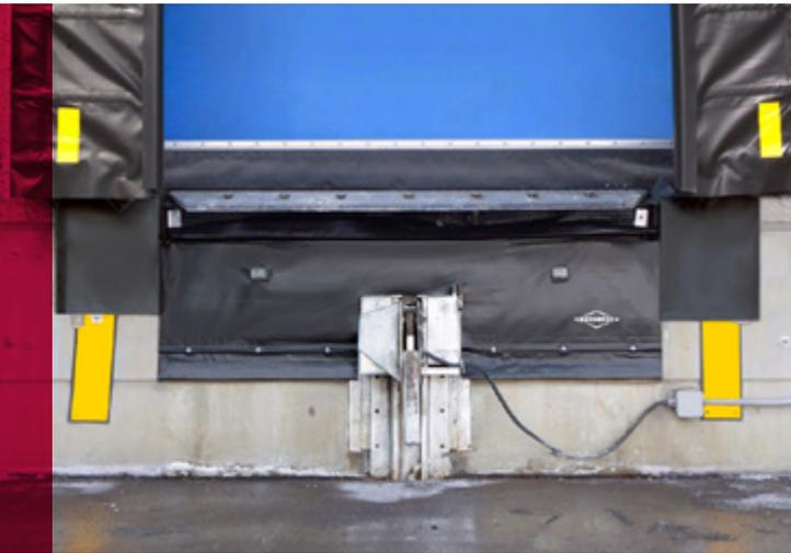
Pit sealed with Rite-Hite® PitMaster Under-leveler Seal.
