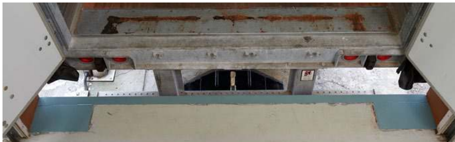
Open gaps between the dock face and trailer allow contamination, infiltration, and increased energy costs
