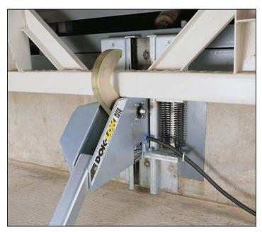
New Belgium installed Dok-Lok vehicle restraints, which have a wide vertical engagement range (9 to 30 inches), helping to prevent trailer separation accidents.
