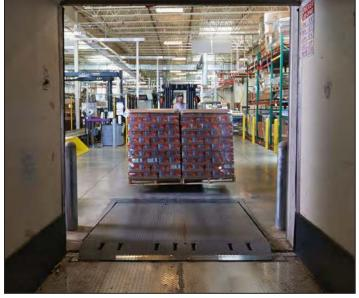
Rite-Hite's hydraulic dock levelers with Smooth Transition technology can reduce "dock shock" by as much as 76 percent when compared to standard levelers.
