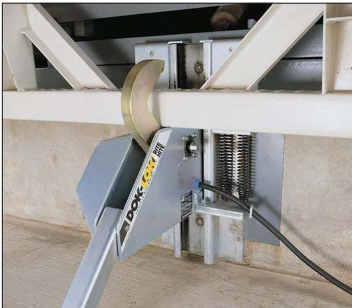
New Belgium installed Dok-Lok vehicle restraints, which have a wide vertical engagement range (9 to 30 inches), helping to prevent trailer separation accidents.
