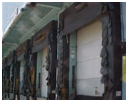
Repeated vertical trailer movement leads to wear on dock seals and bumpers, resulting in higher equipment repair and replacement costs.
