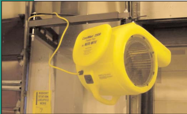
The unique pivoting and swiveling bracketing system of the CoolMan Trailer Fan allows it to service two loading docks.
